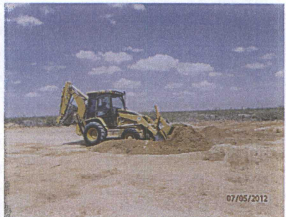
Backfilling site with imported top soil, facing east
