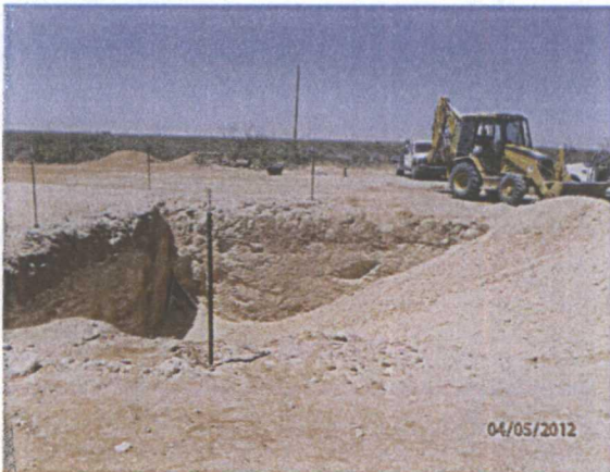
Backfilling site above liner, facing south
