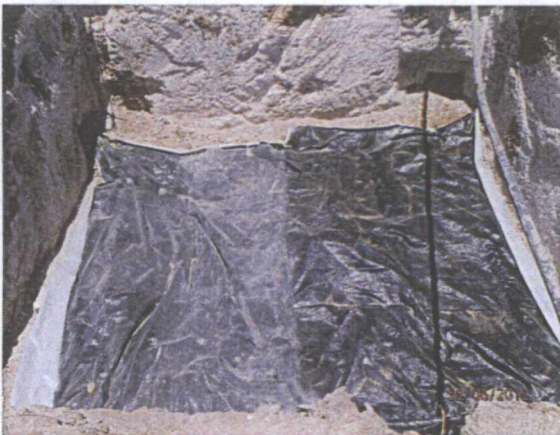
Installing 25'x25' liner at 12' bgs
