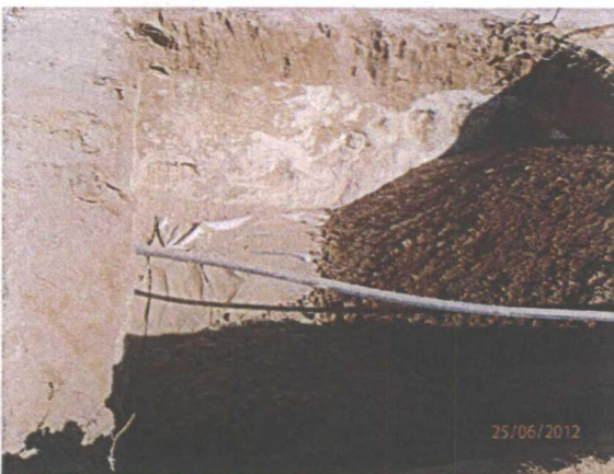
Backfilling site above liner
