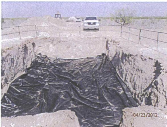
Installing 30x20, 20 mil reinforced liner @ 6' bgs, facing east
