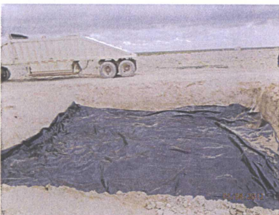
Installing 30x30' 20 mil liner @ 6' bgs, facing south
