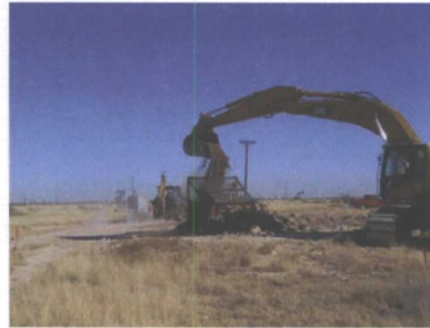
screening the excavated material, facing east 12/8/2010
