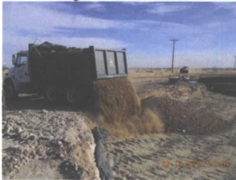
backfilling the excavation 12/20/2010
