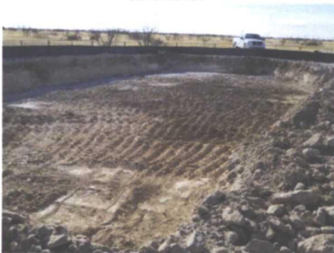
final 80x40x4.5-ft deep excavation, facing southwest 12/10/2010
