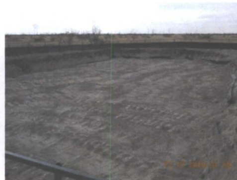
liner padded with 6 inches of imported soil, facing southwest 12/17/2010
