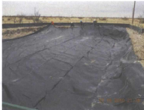
80x40-ft liner being installed, facing southwest 12/17/2010
