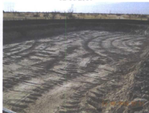
excavation padded with 6 inches of imported soil, facing southwest 12/17/2010
