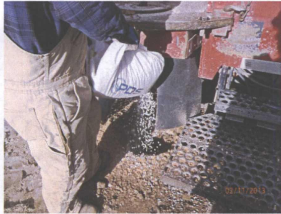
Plugging the soil bore with bentonite 2/11/2013
