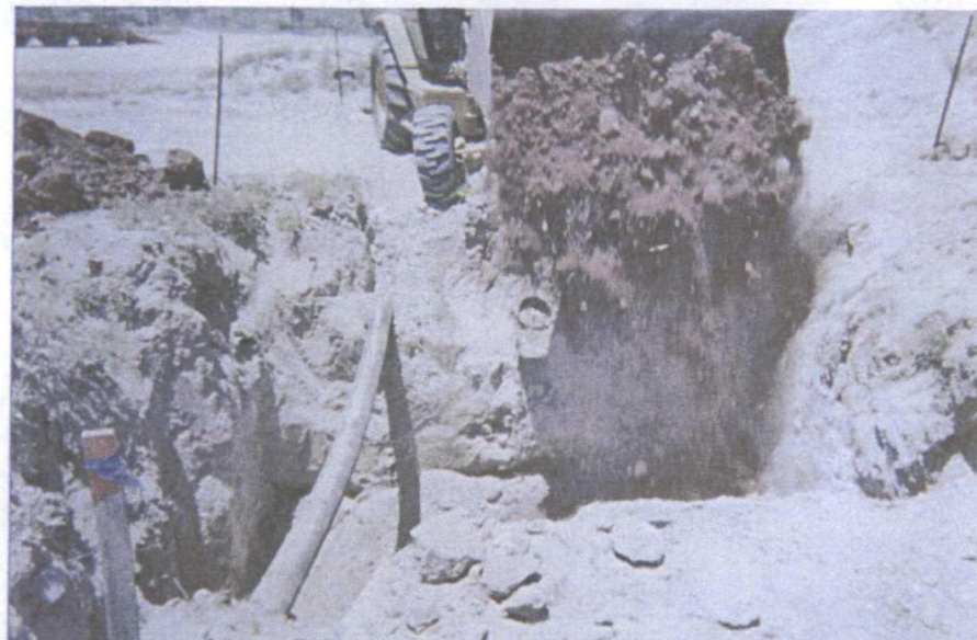
clay barrier being installed
