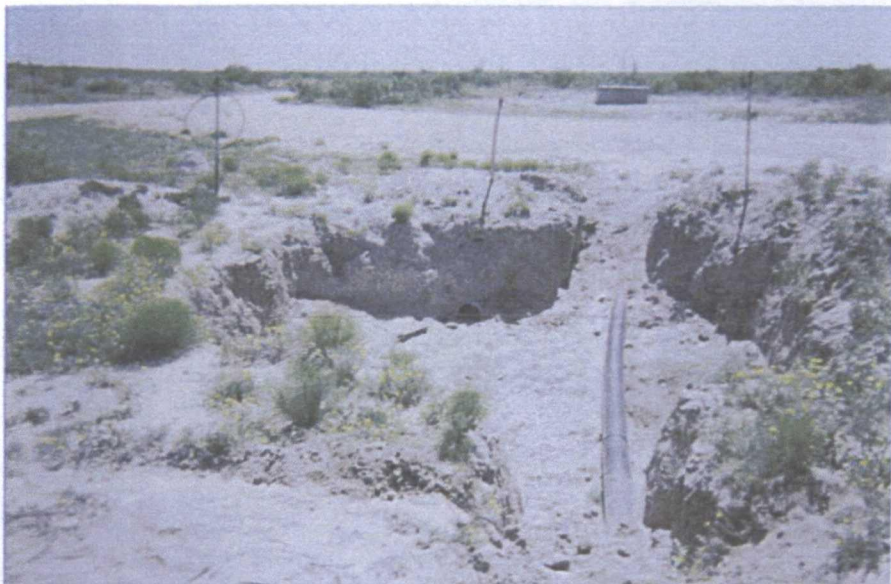
former junction box site in foreground and new, watertight box in background
