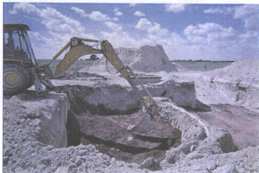
clay barrier being compacted
