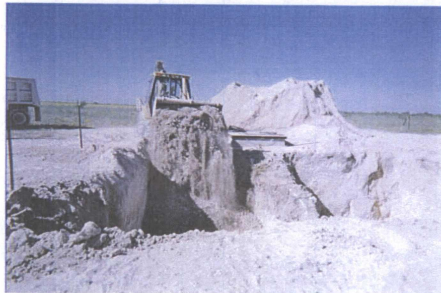
backfilling excavation site up to 5 ft BGS, facing west
