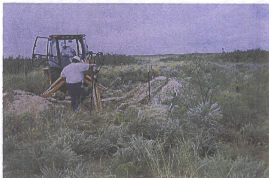
Delineation trench being excavated
