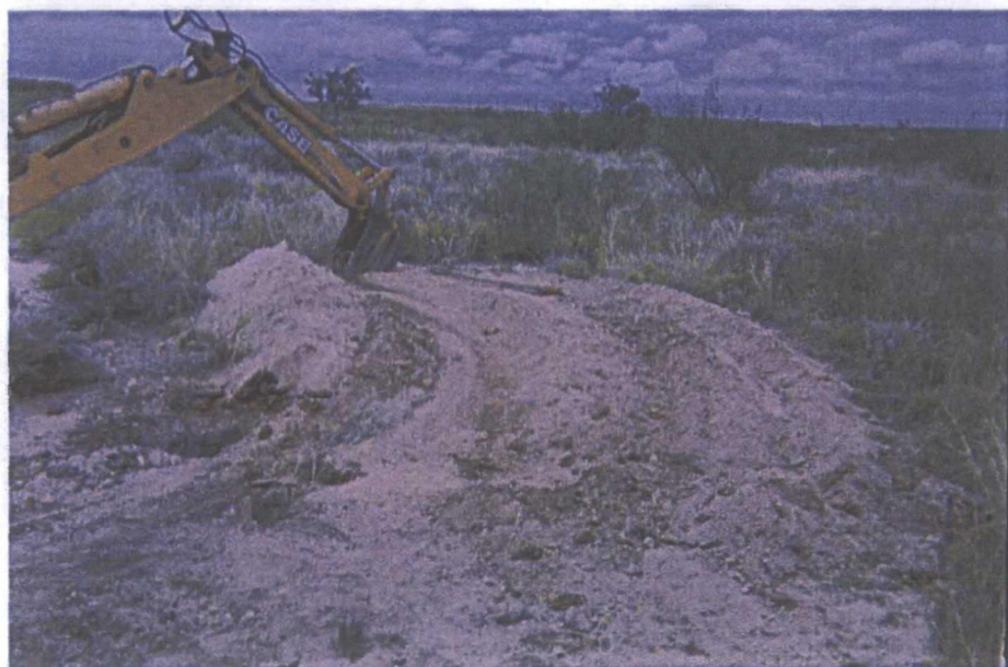
Backfilling excavation
