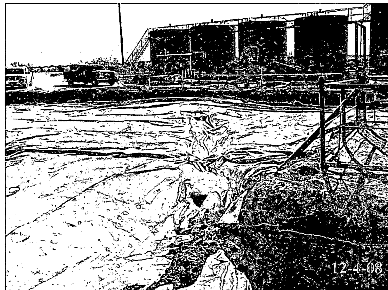
After installation of the 20 mil liner on the location.
