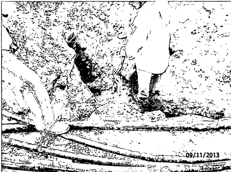
Hand spotting gas line, facing south 9/11/13
