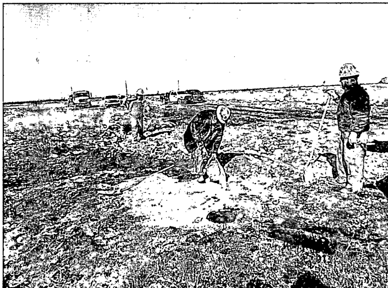
Plugging SB-1 in total with bentonite, facing northwest
