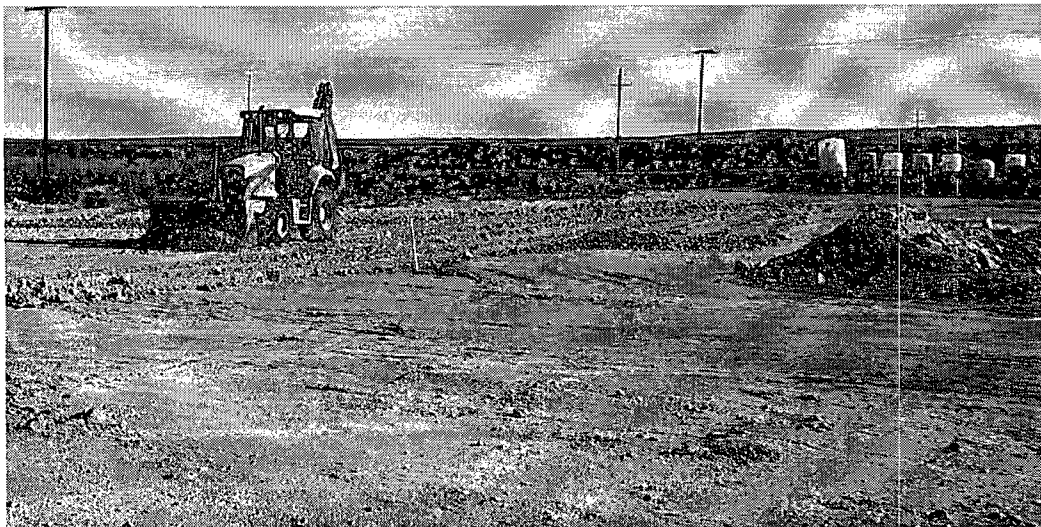
Figure 2: Grading of former containment berms. The former berms were either thin spread on location or placed around location to reinforce existing berms (Figure 3).
