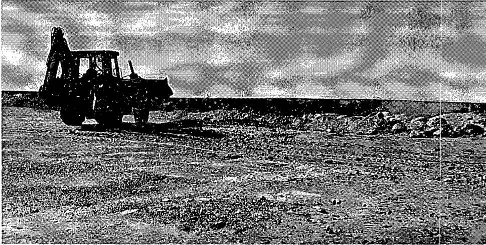
Figure 3: Re-using material from former containment berms from the CleanWave system to reinforce existing containment berms.
