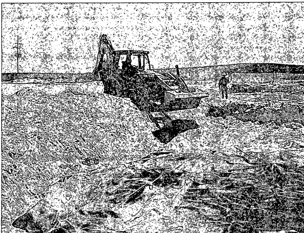
View North – Backfill
