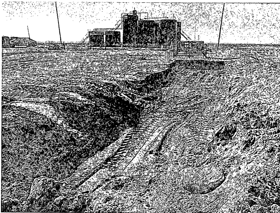
View West – AH-1, AH-3, and AH-5 areas
