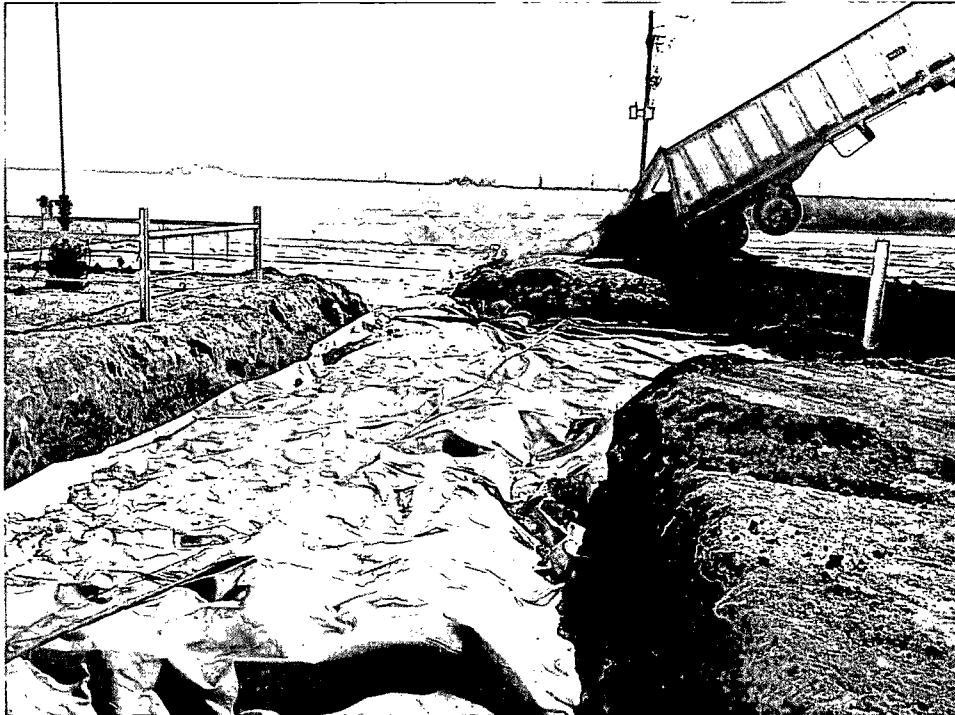
Liner installed in completed excavation, beginning backfill 10/7/13
