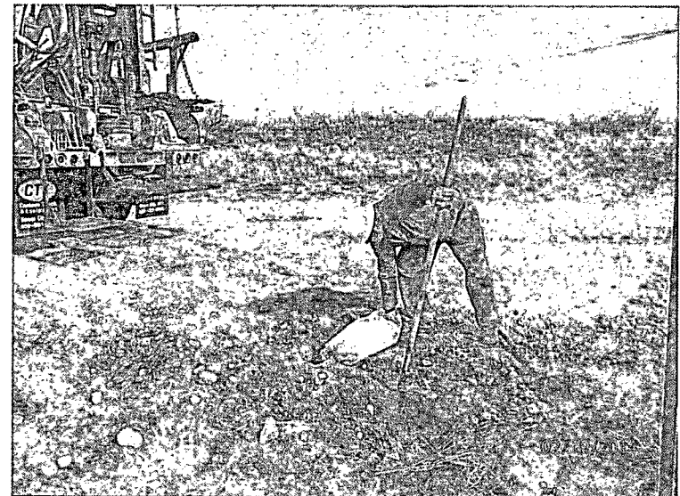
Plugging SB-2 in total with bentonite, facing east 2/19/14
