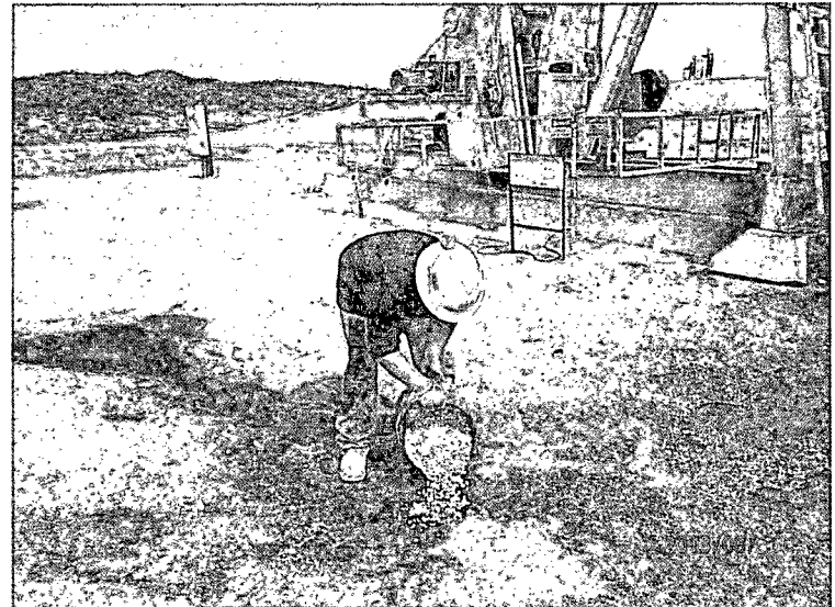
Plugging the augur in total with bentonite, facing NW 8/16/13
