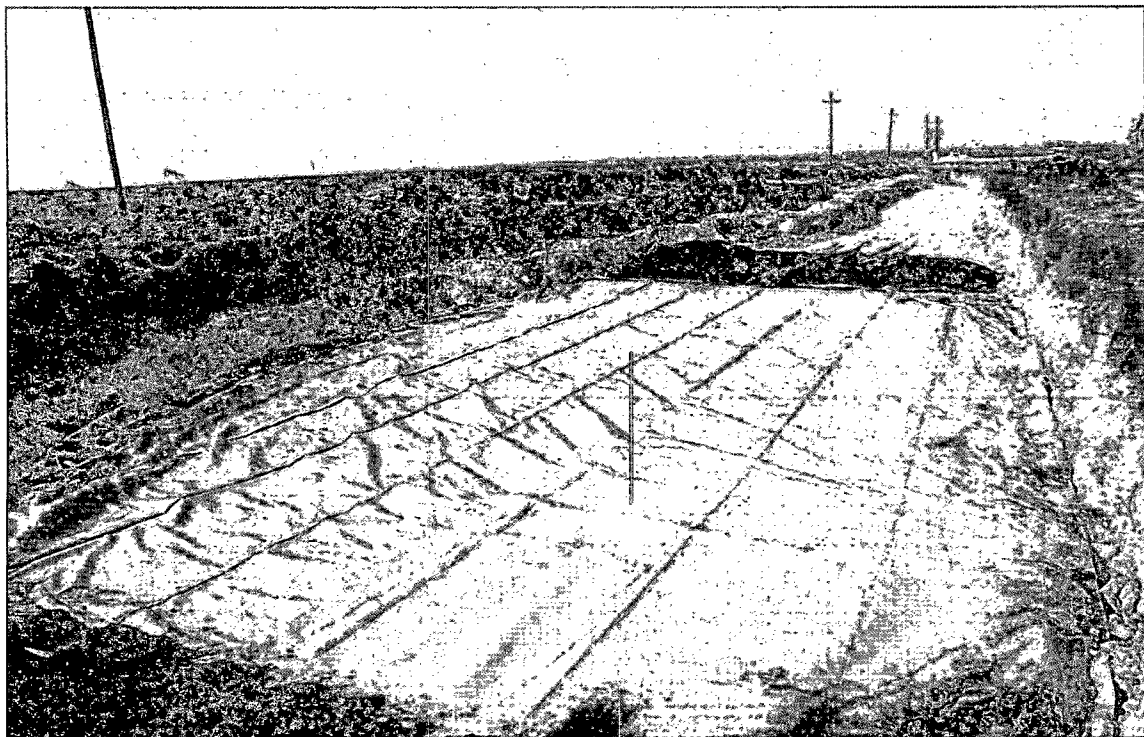
James Ranch Unit #29 SWD - South Excavation, Liner Installation (Looking West)
