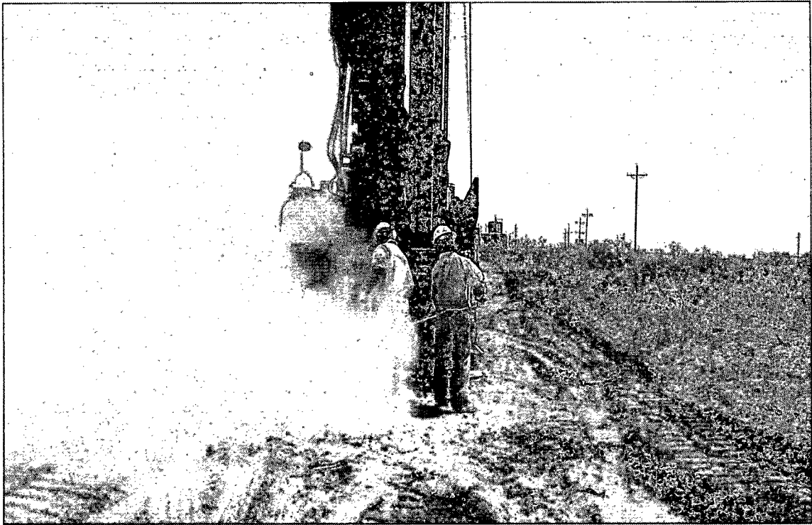
James Ranch Unit #29 SWD - Advancement of Delineation Soil Boring
