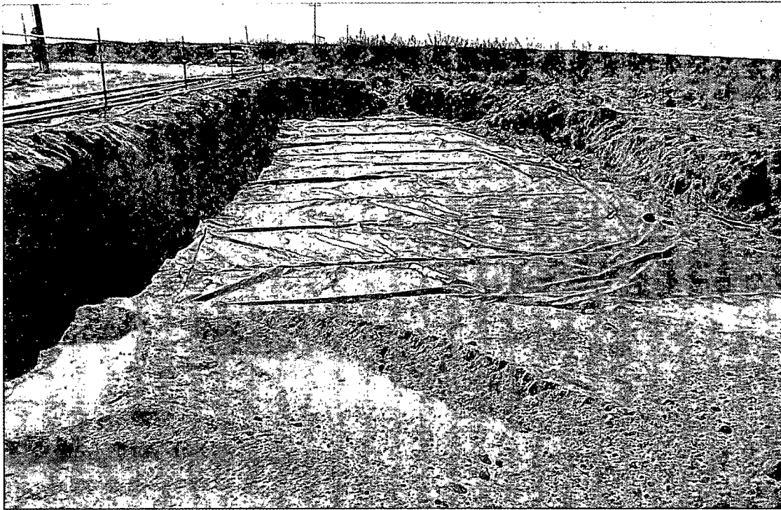
Poker Lake Unit #108 Flowline - Liner Installation, South Excavation
