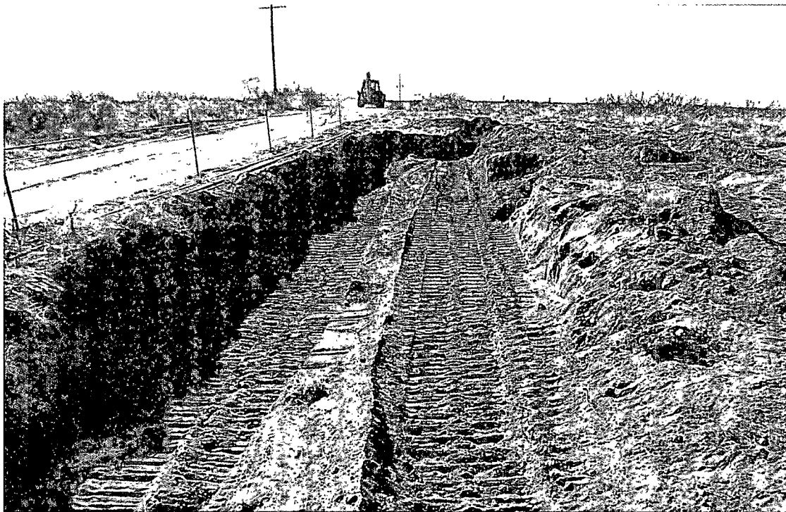
Poker Lake Unit #108 Flowline - North Excavation (Following Installation of Liner & Pad Sand)
