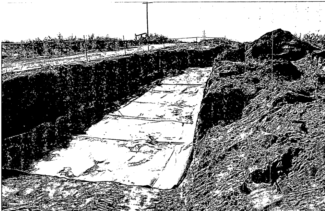
Poker Lake Unit #108 Flowline - Liner Installation, North Excavation
