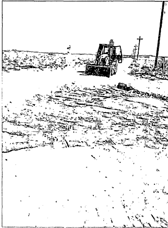
Photograph of backfilling activities at the PLU #154 Flow Line Release Site.
