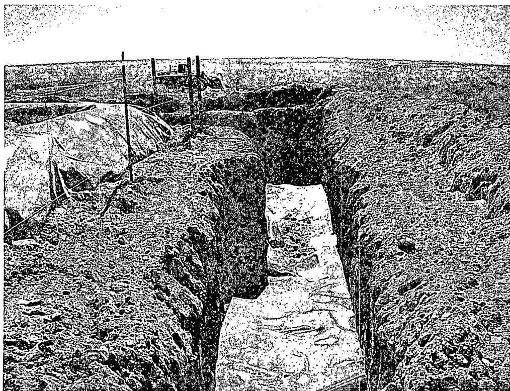
View South – Lined area of T-6, T-7 and SB-3
