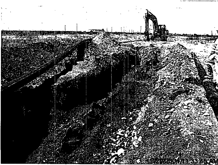
Photo #1: Release area, looking westerly. Note that the steel line is being replaced with a polyethylene line.
