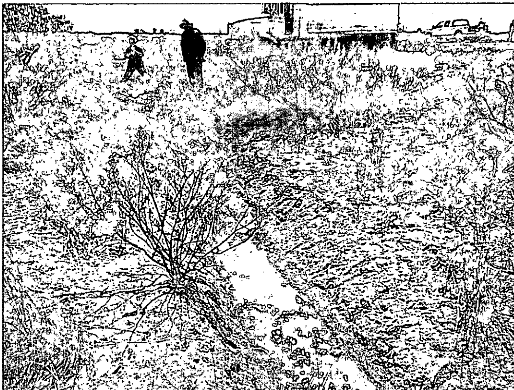
Figure 5. Photograph of the freshwater "Washing" technique utilized to remediate the impacted portion of the ephemeral wash at the Tunstil #1286 Release Site (Looking Northeast)
