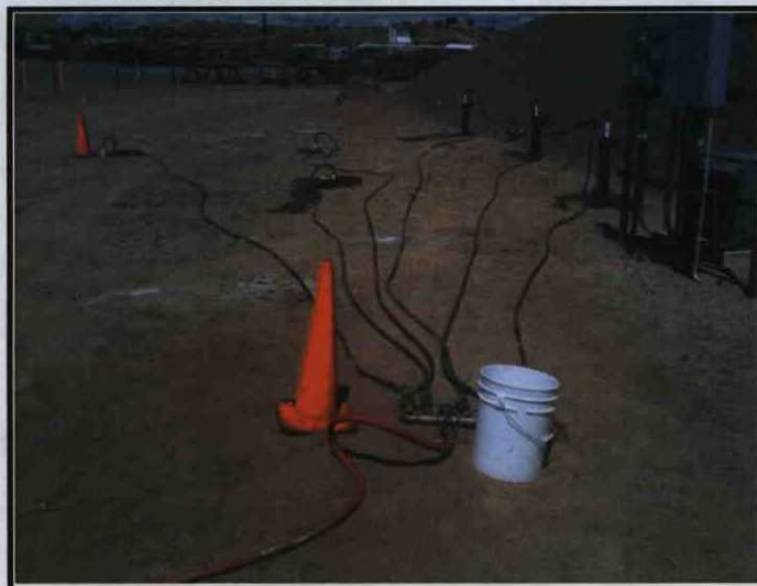
5.) Representative view of the injection of treatment chemicals into select injection points located immediately west of the condensate storage tank containment.
