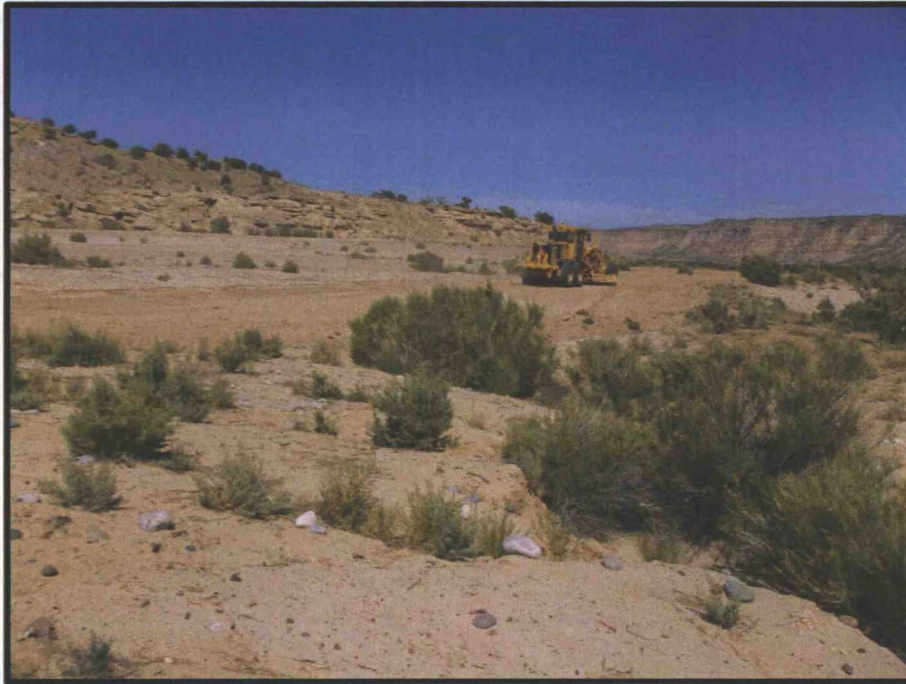
Photo 5: Lower berm contouring during grading activities, southwest section.
