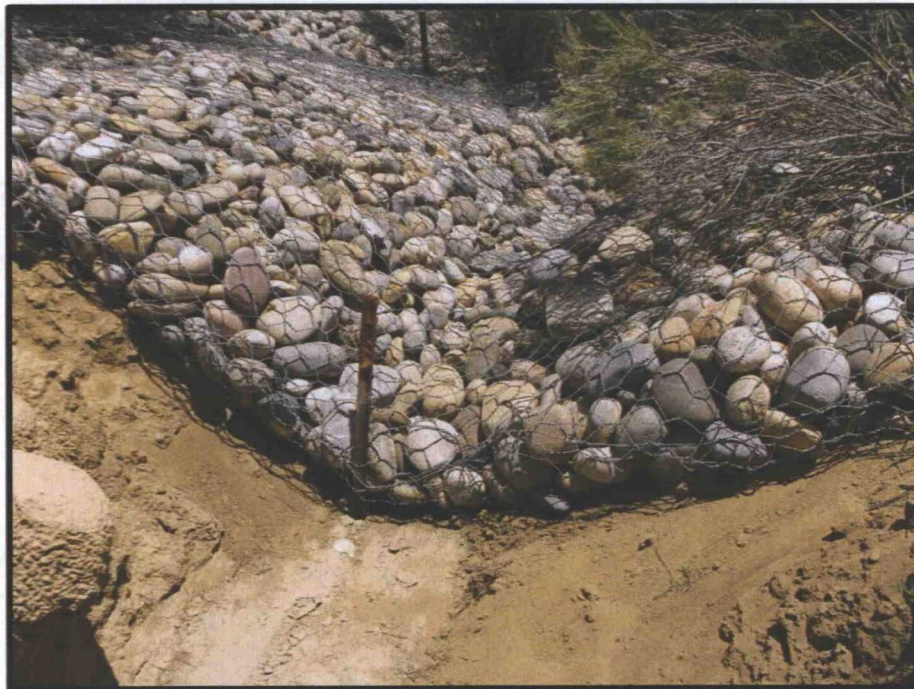
Photo 2: Rip-rap structure sitting on drainage channel (after).
