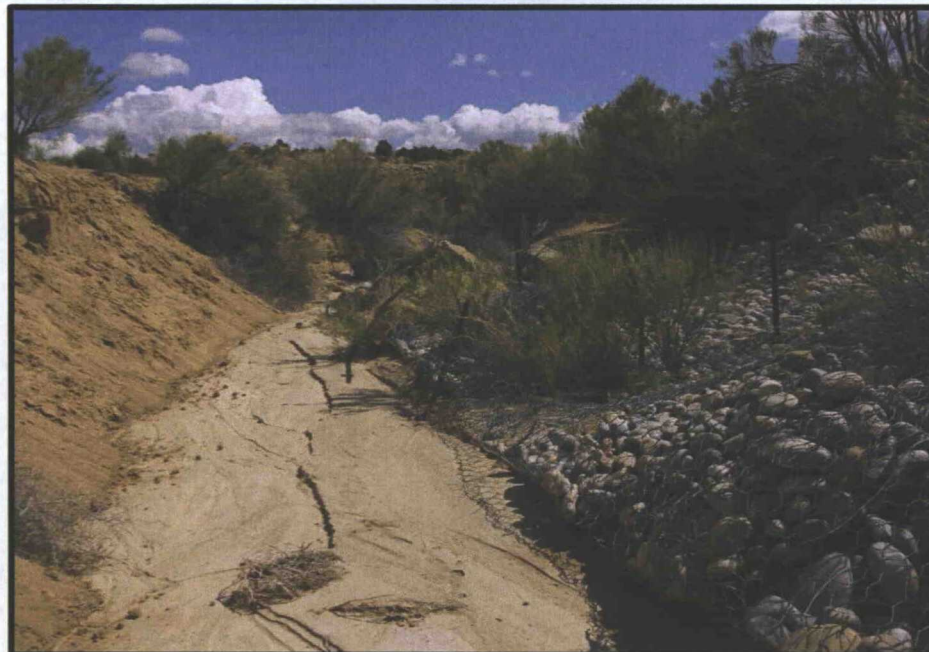
Photo 7: Failure of original stormwater control located in diversion channel west of pond area
