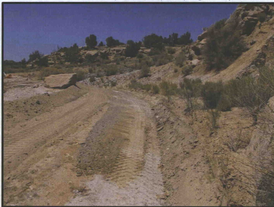
Photo 4: Run-on diversion channel during grading activities, north section.
