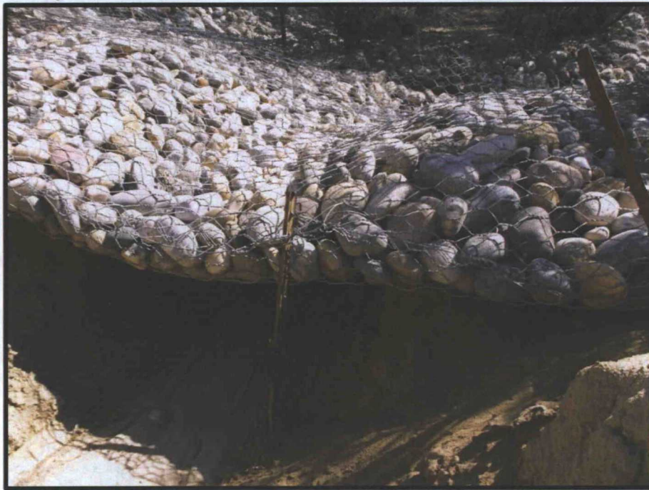
Photo 1: Rip-rap structure above drainage channel (before).
