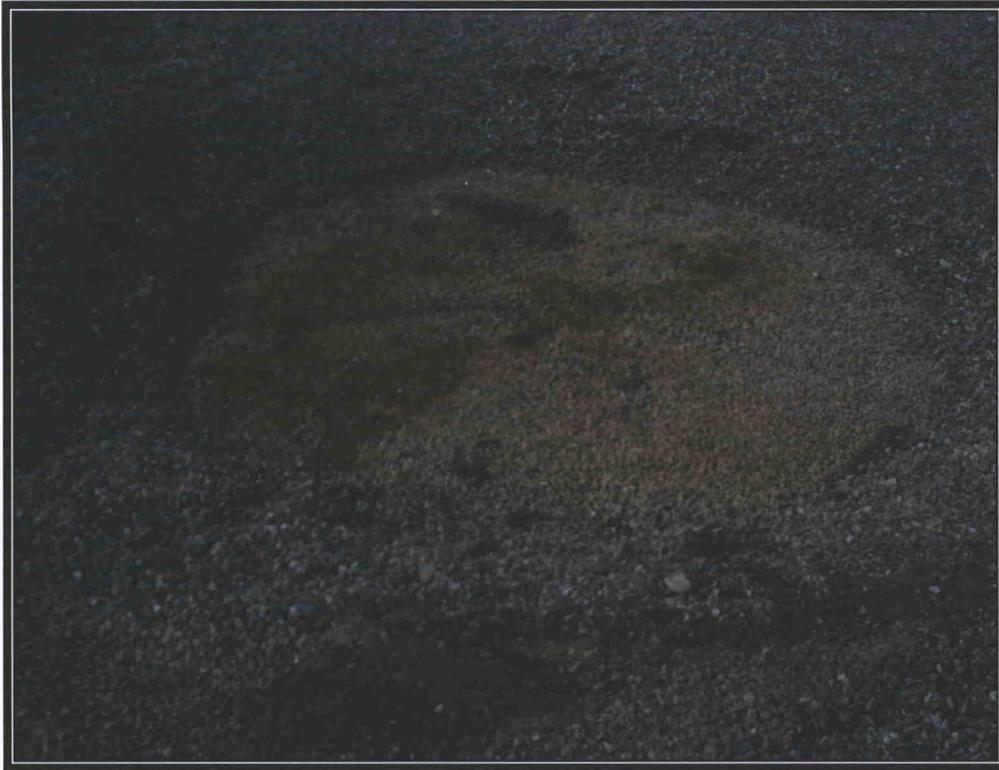
Photo 1: Visible Staining under Aboveground Storage Tank
