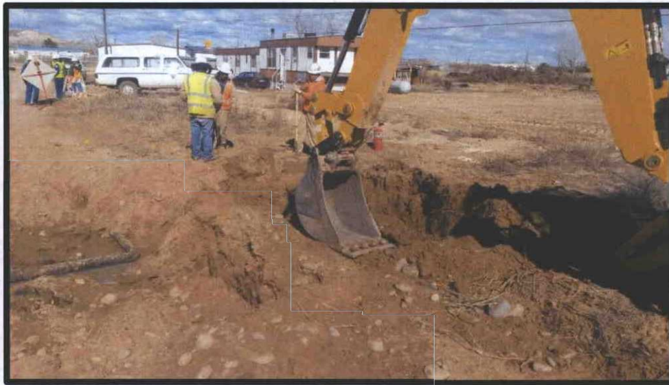
Photo 5: City of Bloomfield waterline, running north parallel to pipeline, marked with yellow flagging. Excavating on the east side of waterline to determine extent of contamination.
