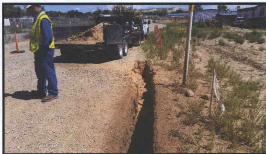
Photo 4: Trench along the waterline completed and backfilling with imported material.
