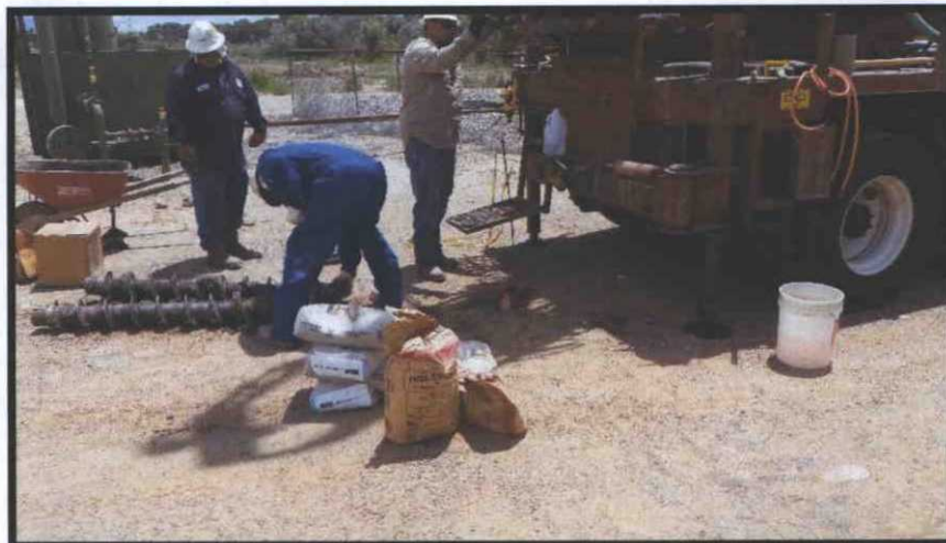
Photo 5: Hollow stem auger drilling method was used to advance the hydro excavated holes to a total depth of 10 feet bgs.
