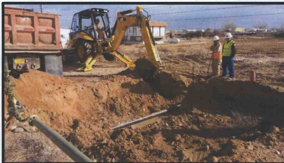
Photo 3: Contaminated soil was placed directly into dump truck for proper disposal.
