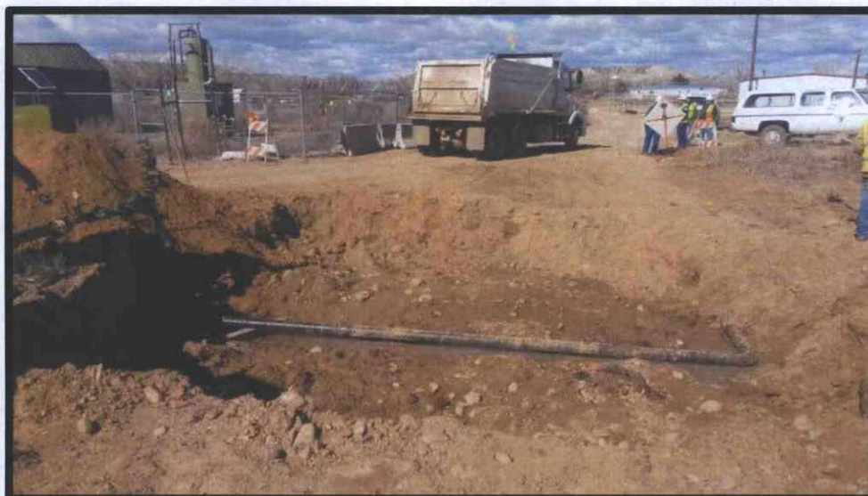
Photo 4: 90 degree bend in pipeline heading north down County Road 5008 visible in right side of photo, view is to north. Also visible is the encountered subsurface water.
