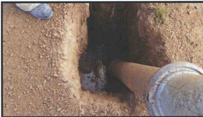
Photo 3: Exposure of the 6 inch PVC waterline in the vicinity of the Masden Gas Com #1E release point.
