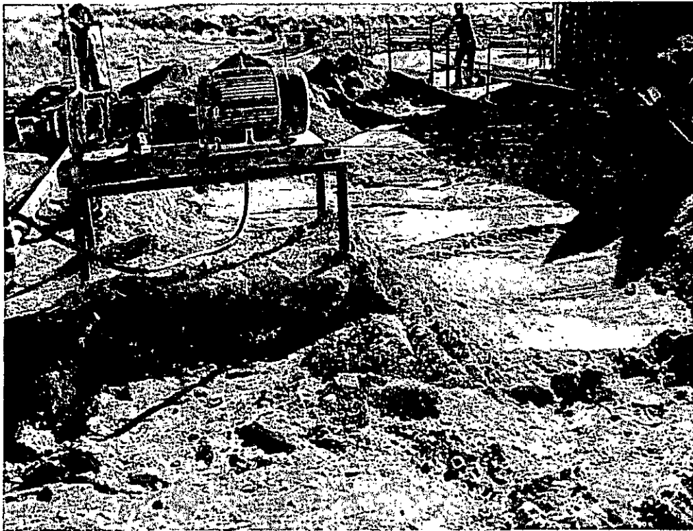
Excavation near SB-2
