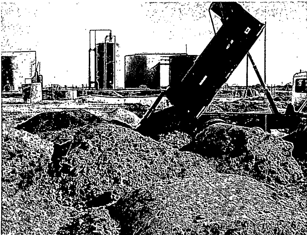
Backfilling with clean material
