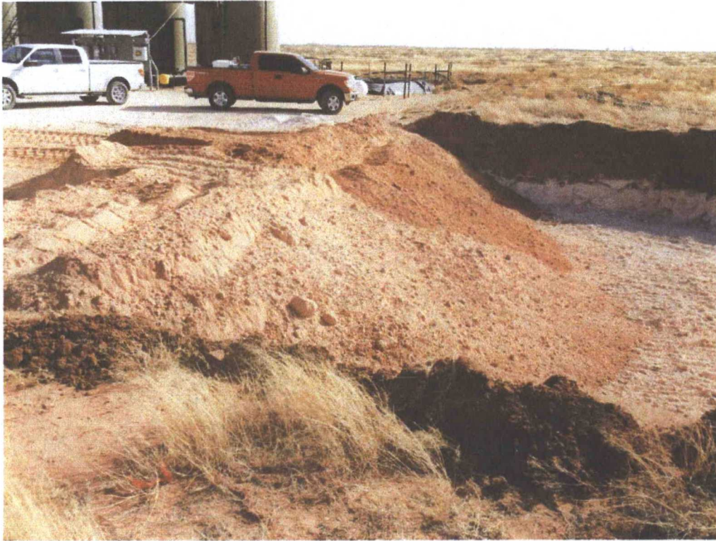
View South – Backfill of AH-1.
