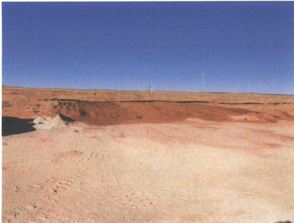
View West – Backfill of AH-1, AH-2, AH-3 and AH-4.
