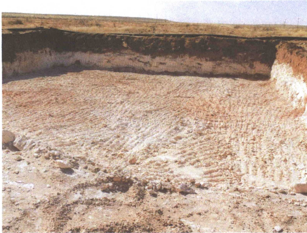
View West – Excavation of AH-1.
