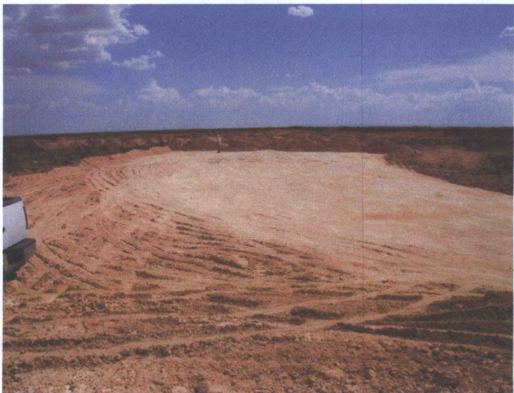
Pasture area lined and backfilled with clean material
