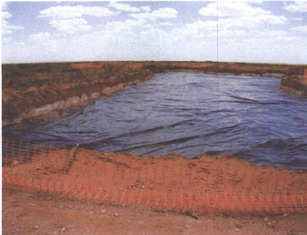
Pasture area - excavation and liner installation
