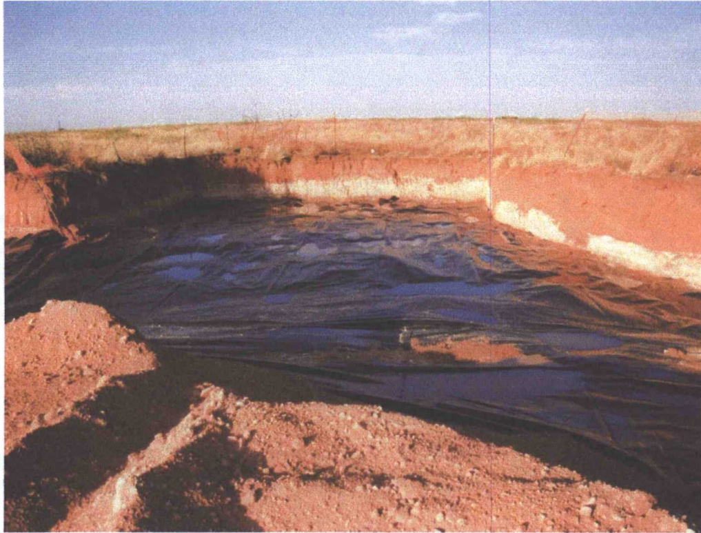
Site excavation and liner installation
