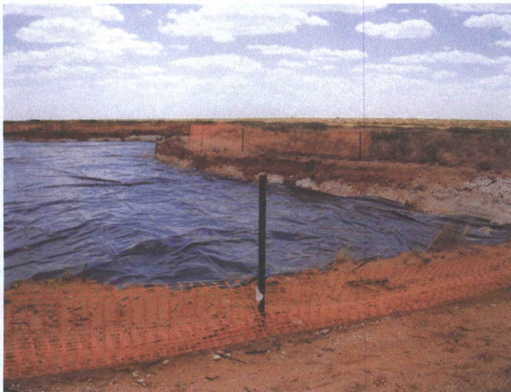
Pasture area - excavation and liner installation
