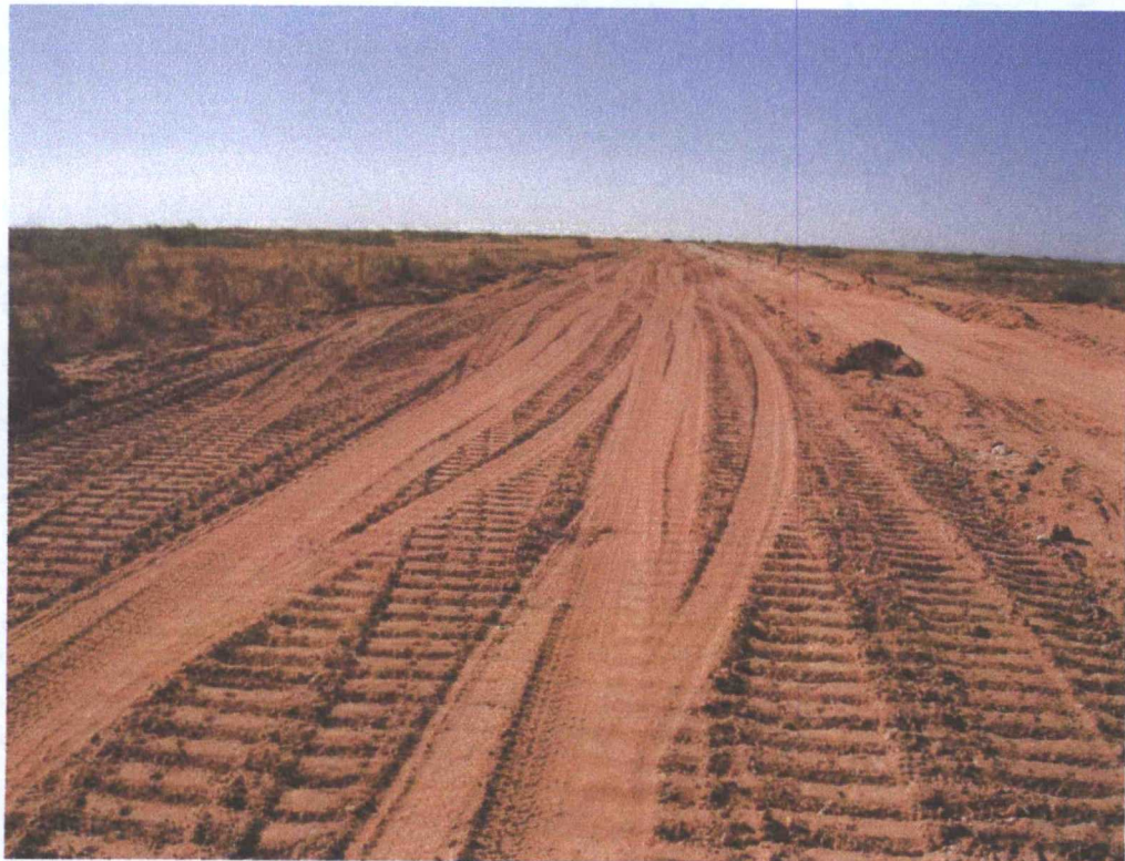
Excavated area backfilled
