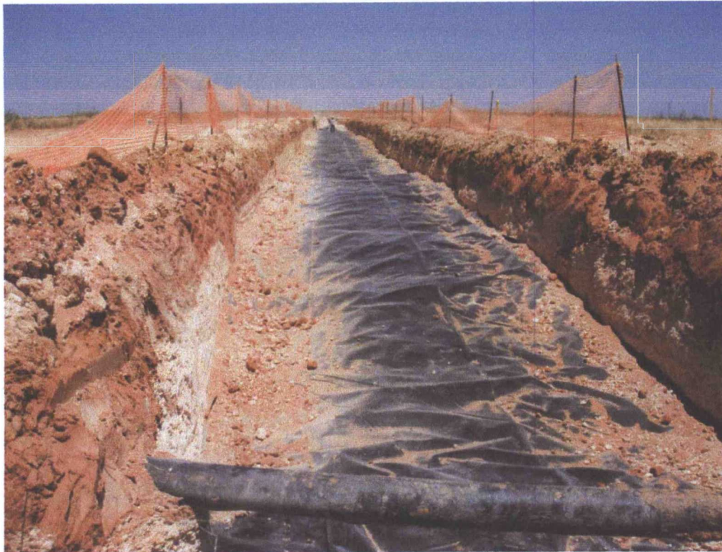
Excavation and liner installation
