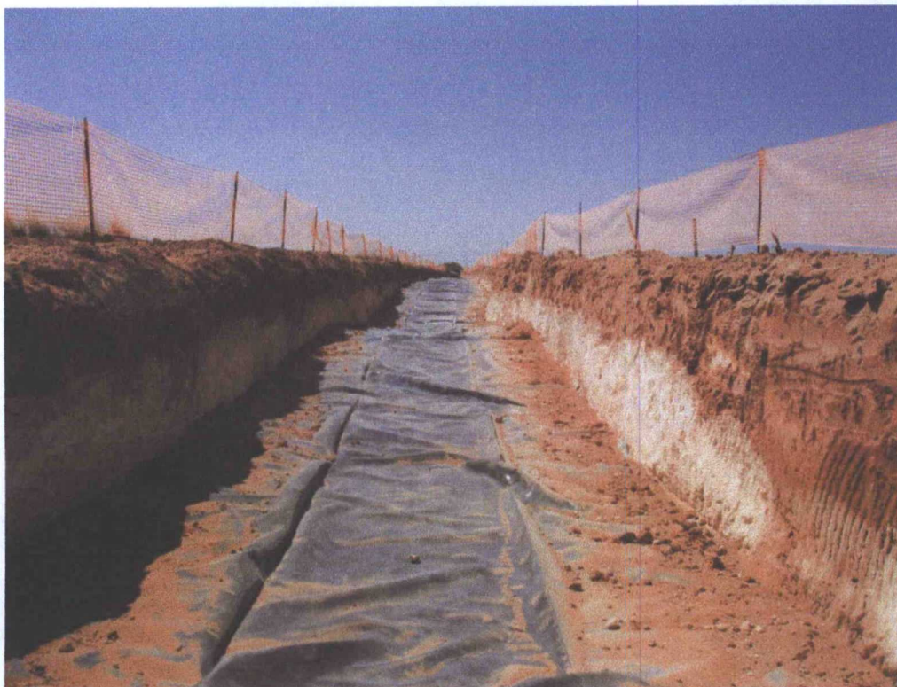
Excavation and liner installation
