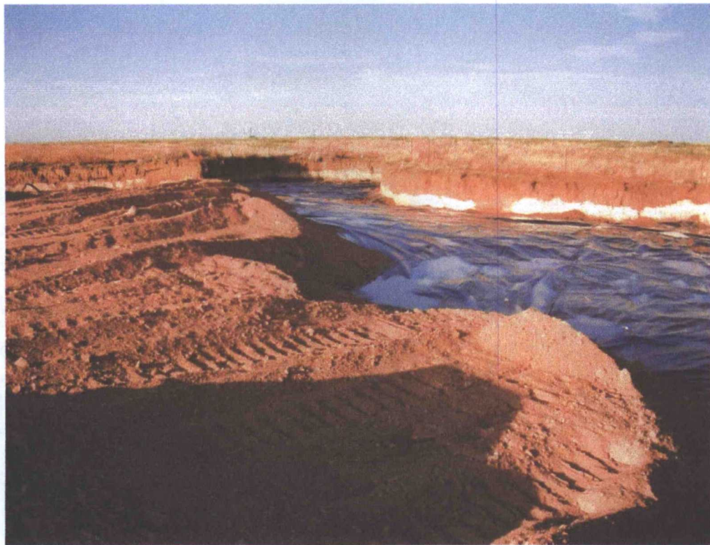
Pasture area - excavation and liner installation
