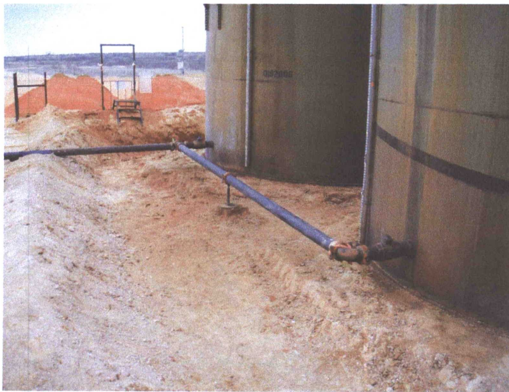
View North – Area of AH-1
