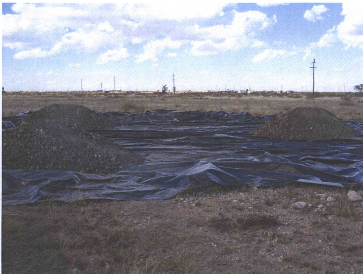
Photo 2. Impacted area after placement of 20 mil poly liner.
