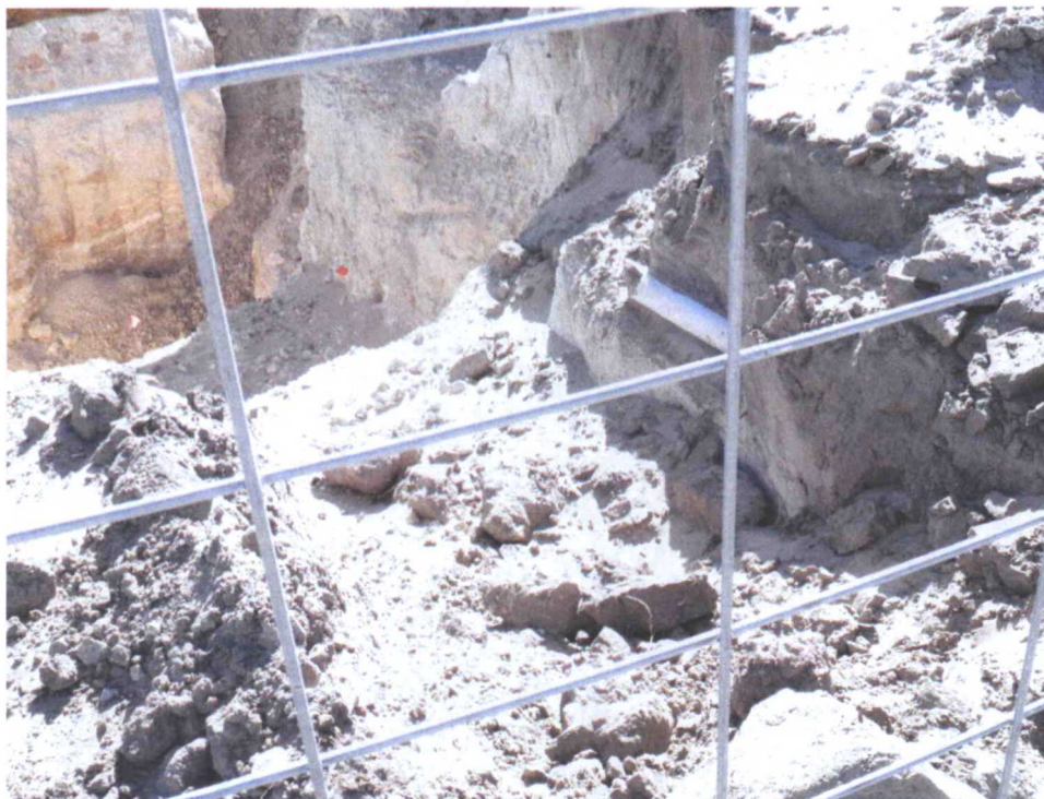
Produced Water (PVC) Line Exposed on North Side of Excavation, March 2, 2011
