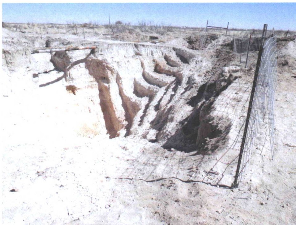
West Excavation after Benching Viewing Northeast, March 2, 2011
