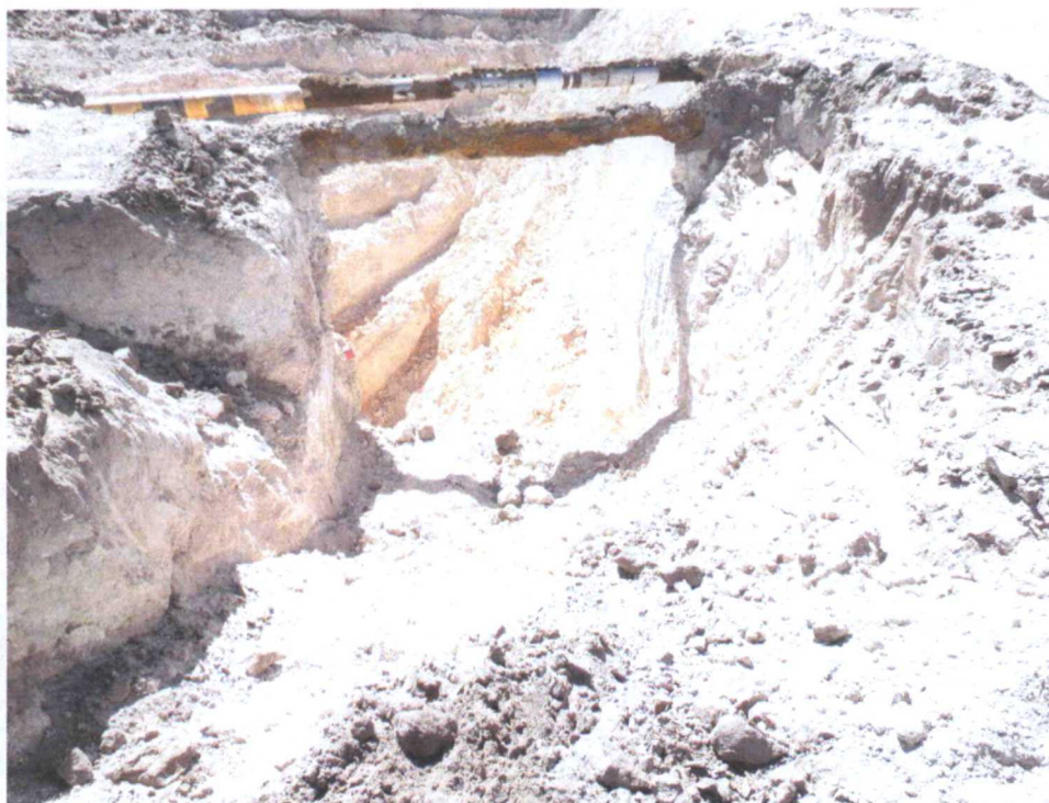
West Excavation after Benching Viewing South, March 2, 2011
