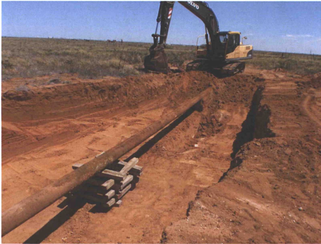
Excavation activities at the Line 4A Release Site. (Looking South)
