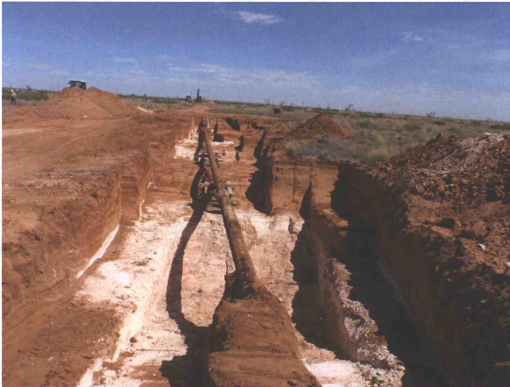
Excavation activities at the Line 4A Release Site. (Looking North)
