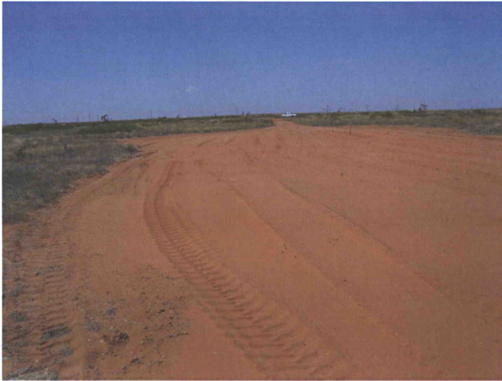
Backfilled excavation at the Line 4A Release Site. (Looking North)
