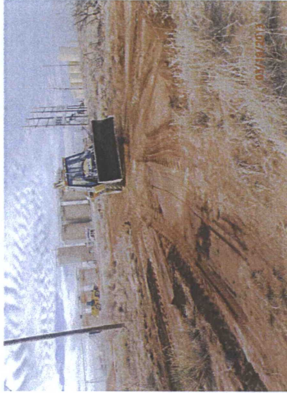
Scrape completed to 1', facing southeast
