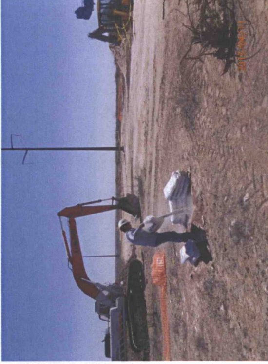
Plugging temporary MW in total with bentonite, facing southeast 4/11/13
