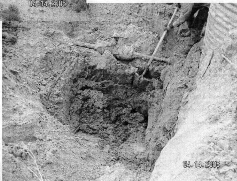
Obvious hydrocarbon contamination beneath the line leak
