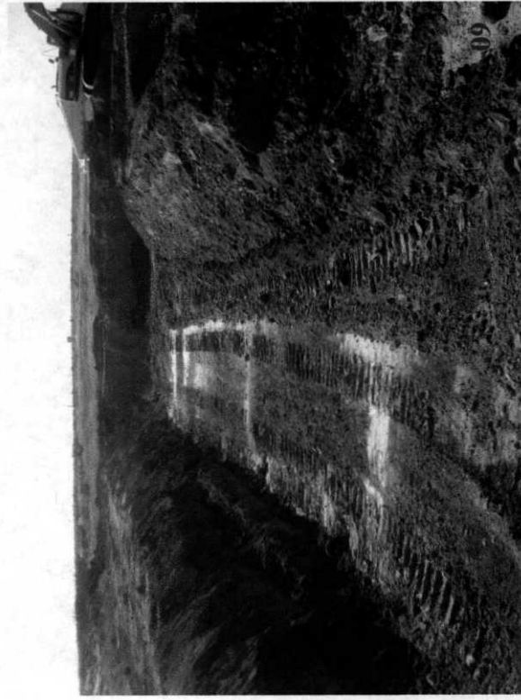
TP3 and TP4 after removal of drilling mud and liner at 8' bgs.
