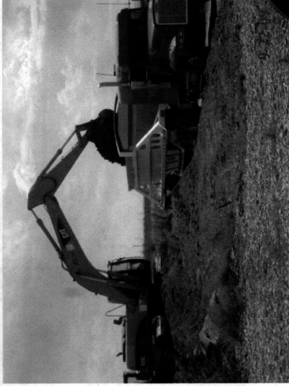
Loading drilling mud on trucks for disposal.
