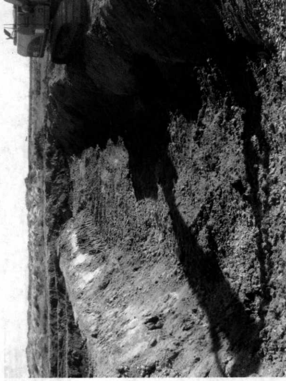
TP1 and TP2 after removal of drilling mud and liner at 8' bgs.
