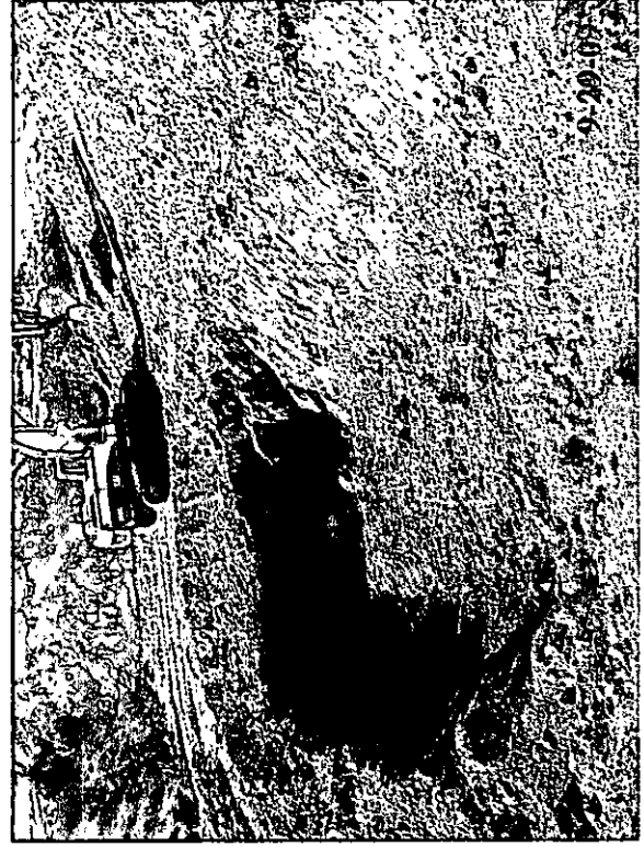
TP5 after excavation of impacted soil to 20' bgs.
