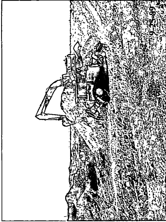
Excavating impacted soil underlying the pit area.
