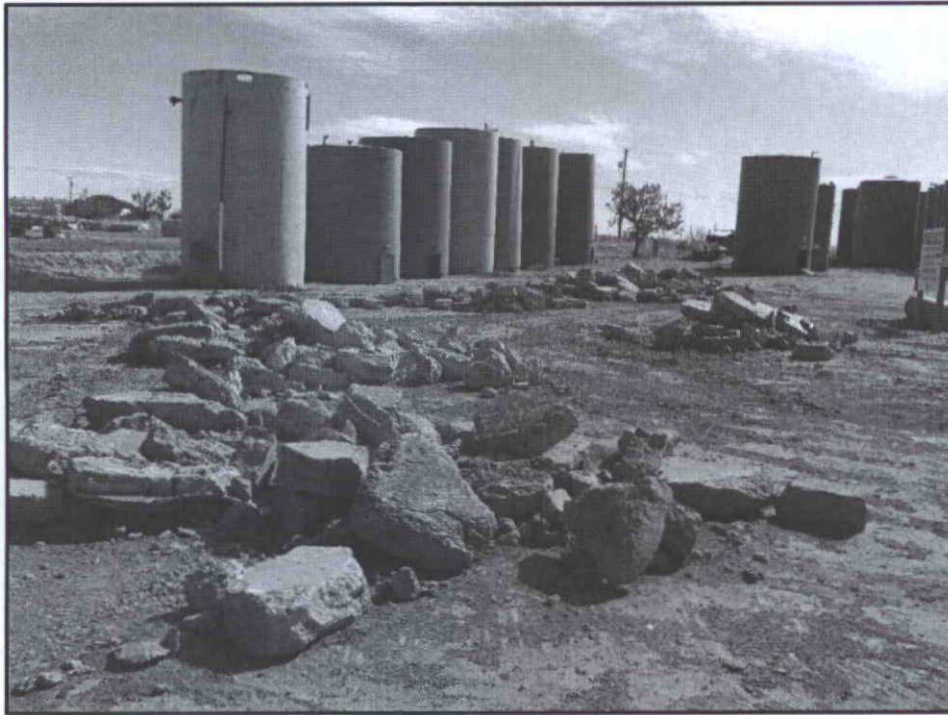
Photo 3: Concrete debris layed out in segements representing each wall and floor section during the third concrete sampling event on March 31, 2014.
