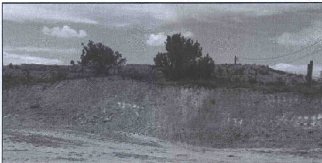
Photo 7: View of the borrow area where virgin soils were obtained for backfill, just southeast of the concrete impoundment location.
