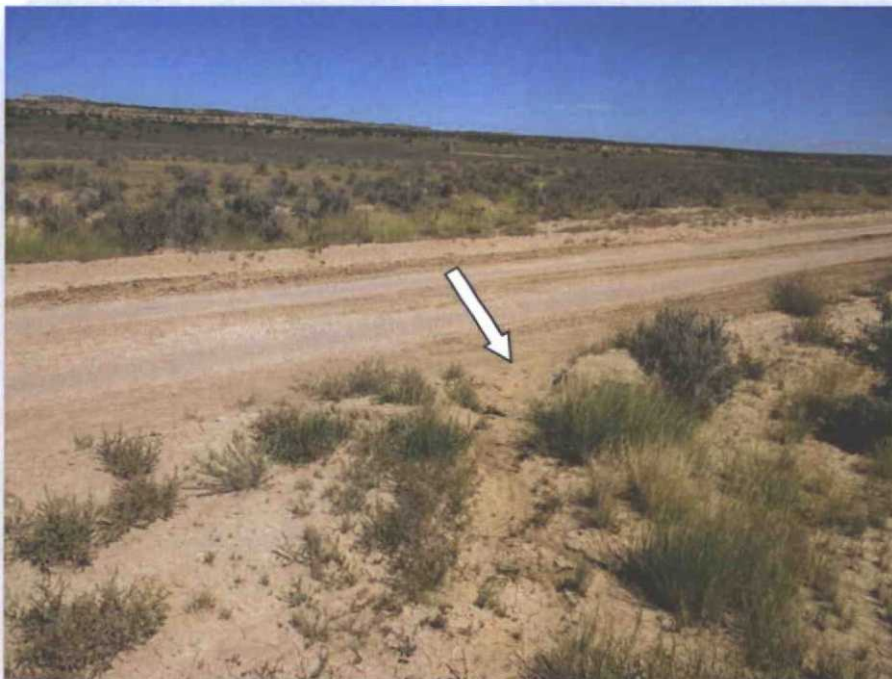
Figure1. Silted-in culvert at Area 1
