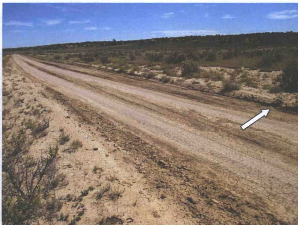
Figure 3. Area 1 - Drainage entrance at road, with no clear outlet
