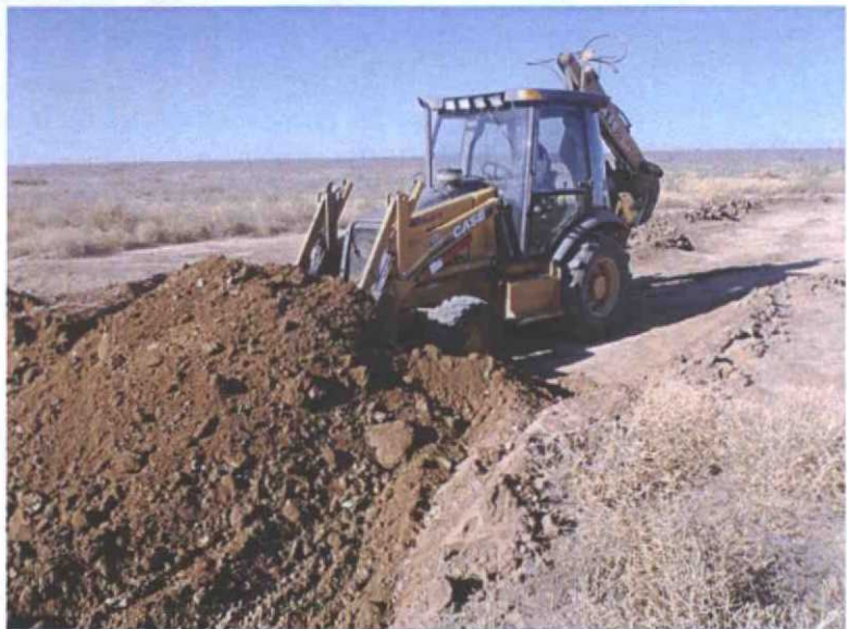
Excavating, facing southwest
