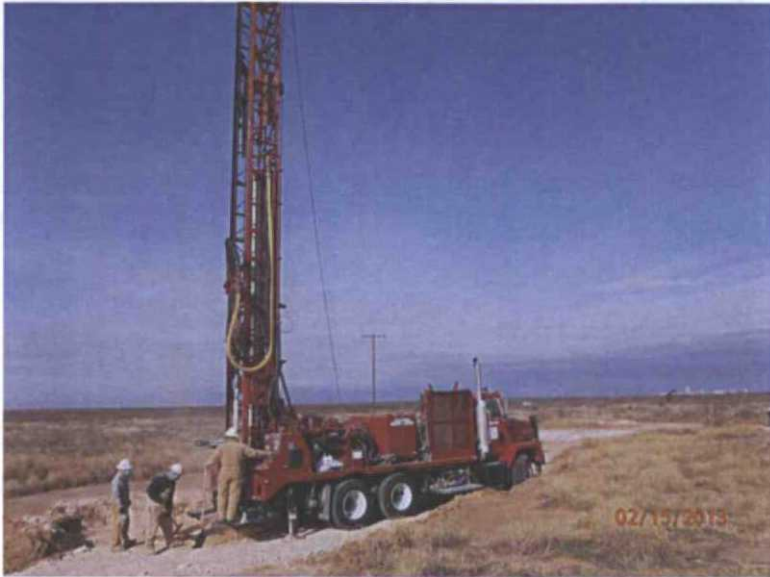
Installing SB-1, facing west
