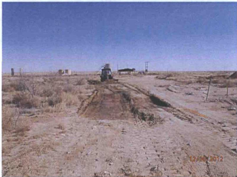
Excavating, facing east
