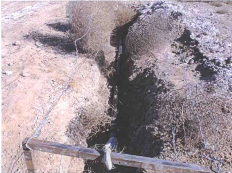
Release source, facing east
