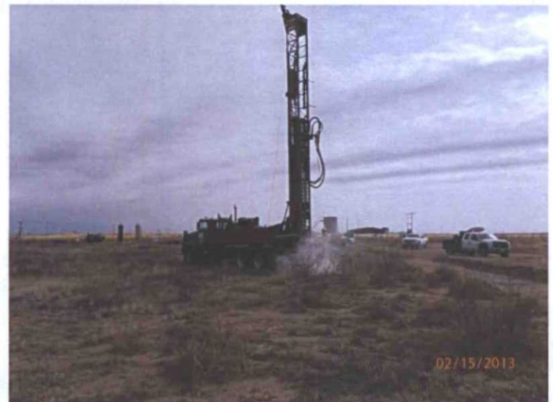
Installing Temp MW, facing east
