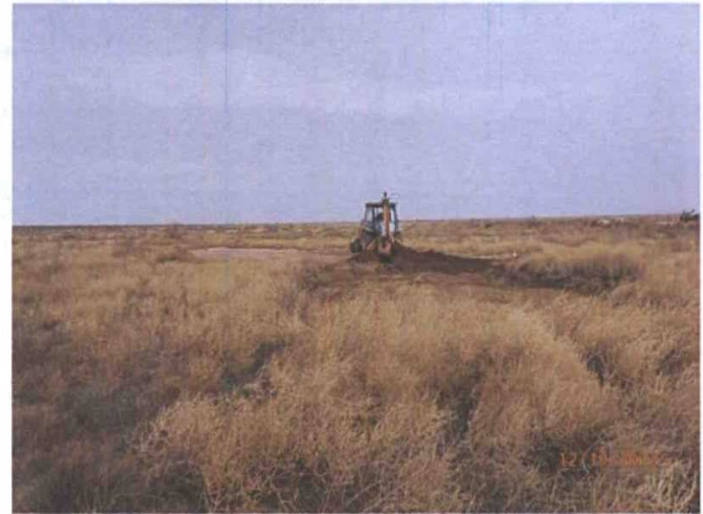
Excavating, facing north
