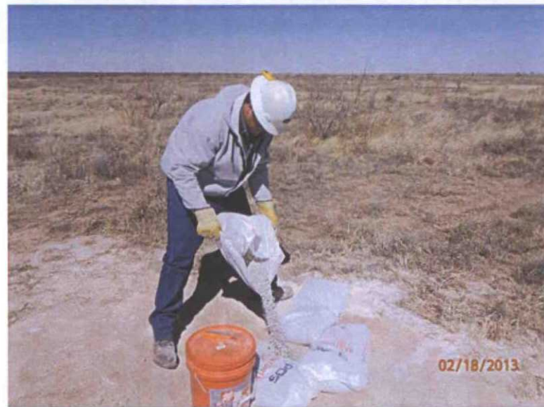
Plugging Temp MW in total with bentonite 2/18/13
