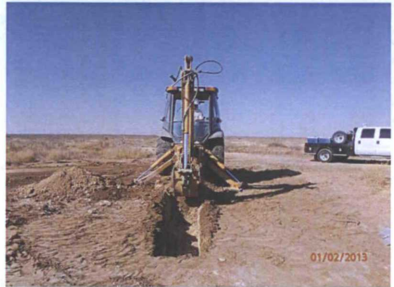
Digging vertical #2, facing northwest
