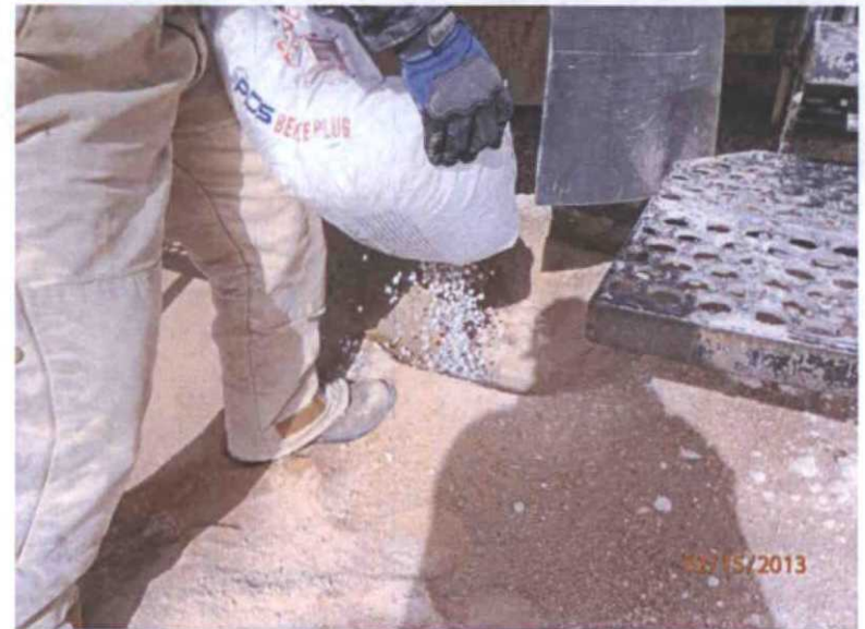
Plugging SB-1 in total with bentonite
