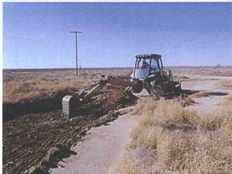
Excavating, facing west
