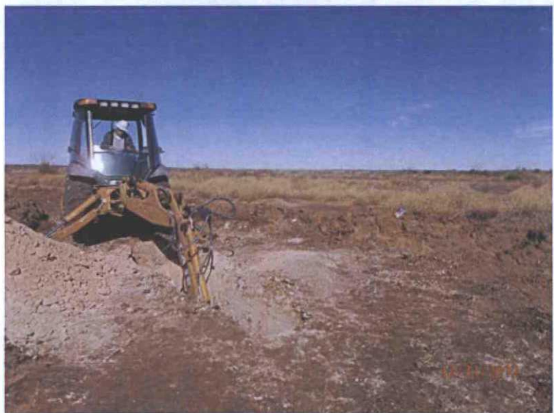
Digging Vertical #1, facing north
