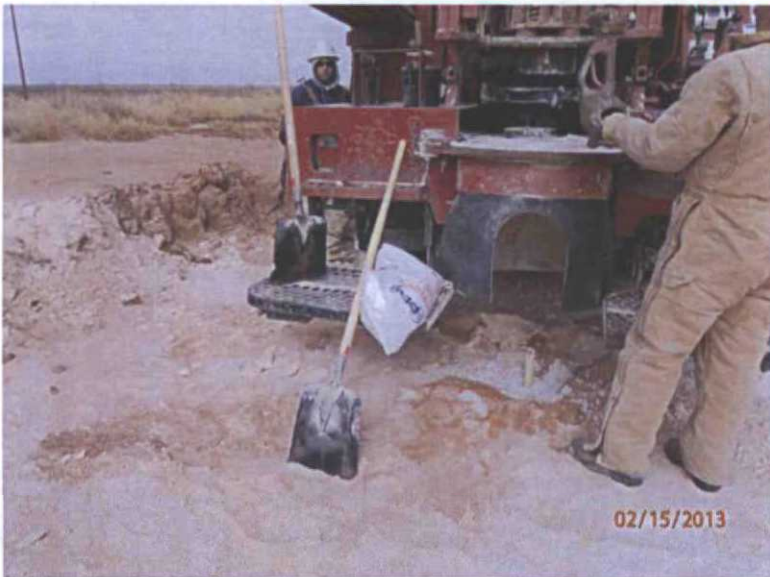
Completed SB-1, facing north
