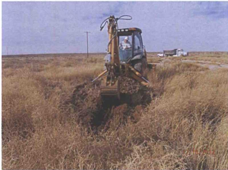
Excavating, facing north
