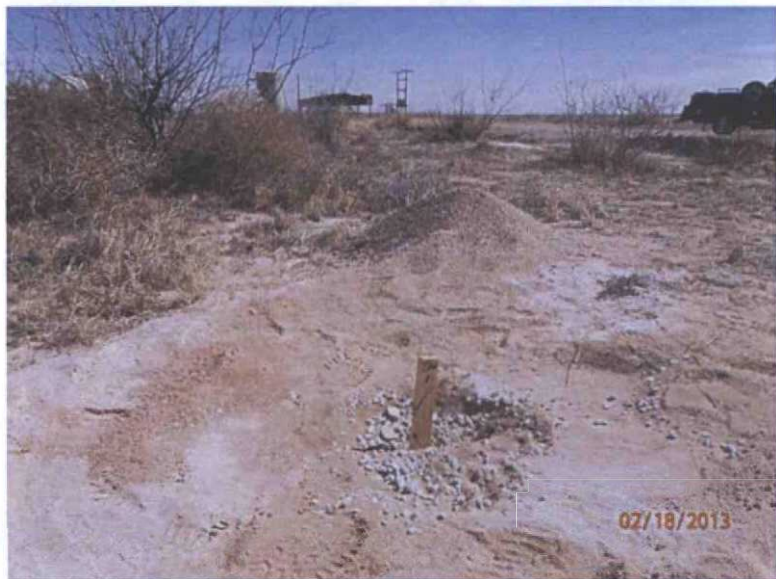
Completed Temp MW, facing east 2/18/13
