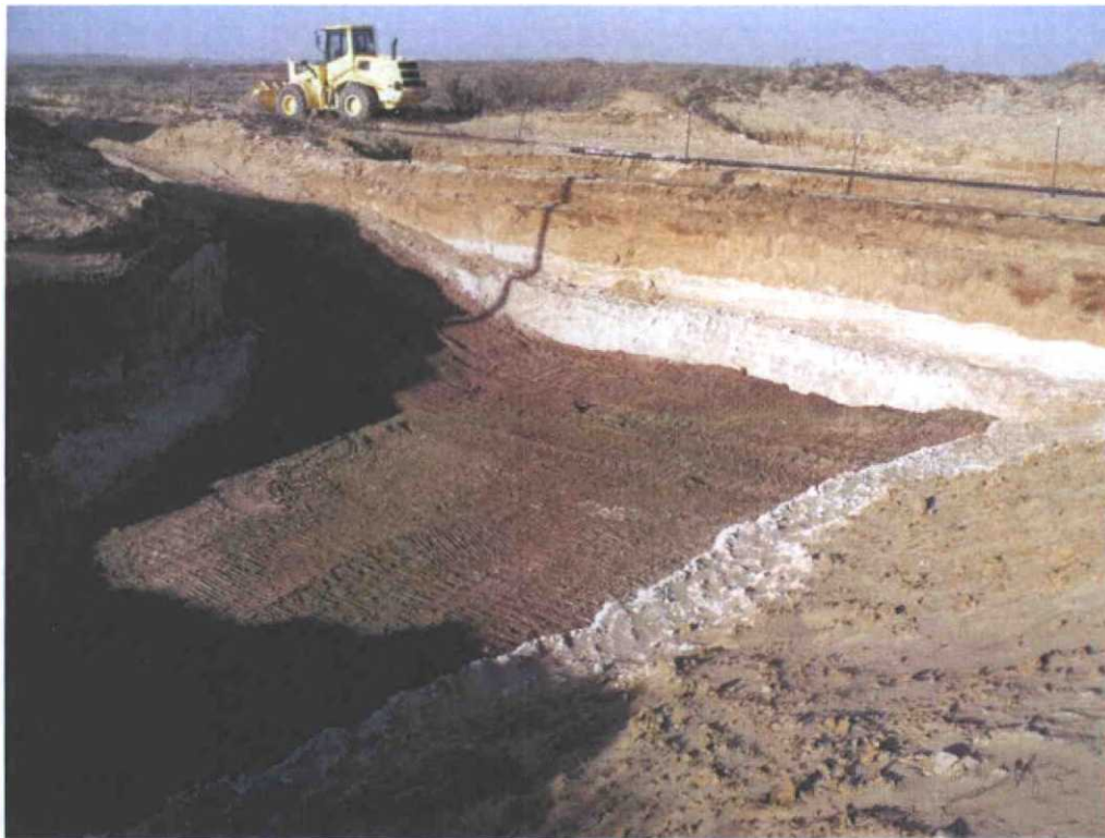
Photograph No. 7 – Looking westerly at two (2) feet thick clay barrier
