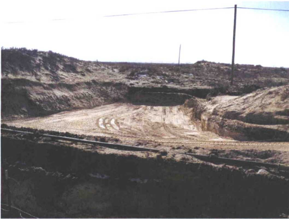
Photograph No. 8 – Looking southerly at finished sub-surface grade in preparation for advancement of soil borings
