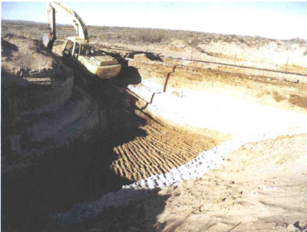
Photograph No. 6 – Looking westerly at finished bottom of South excavation awaiting clay barrier
