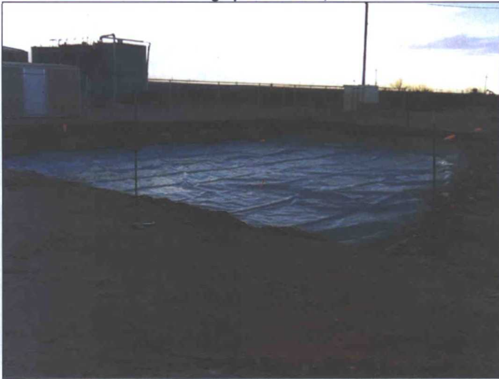
20 mil liner bottom hole of excavation facing southeast
