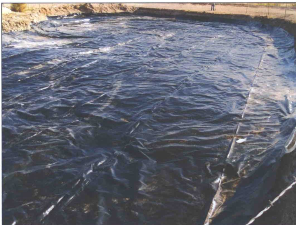
Middle of excavation with liner
