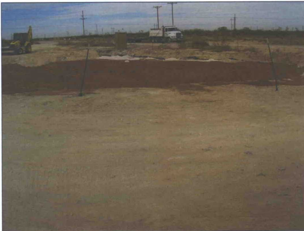
Backfill topsoil and caliche mix
