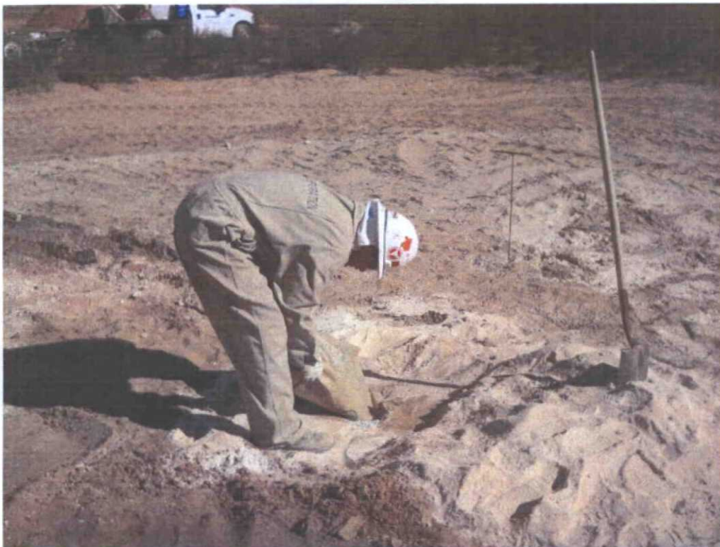
Photograph of the installation of bentonite plug in SB-1 at the Trunk MA-4 #105 Release Site.
