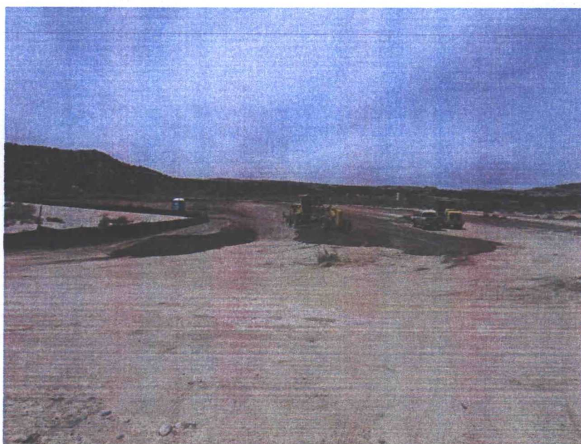
Photo 7 Grader Spreading and Contouring
