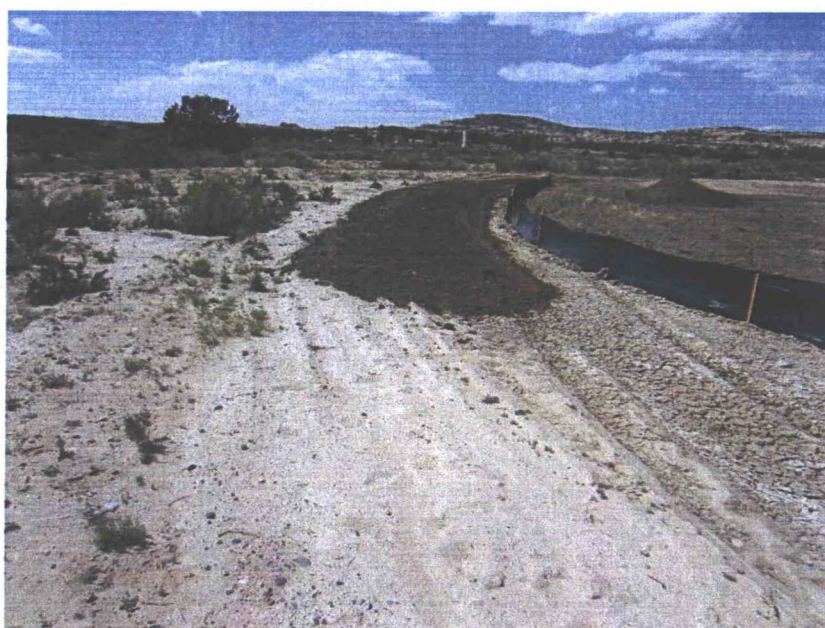
Photo 8 Soil Cap Below Down Gradient Berm
