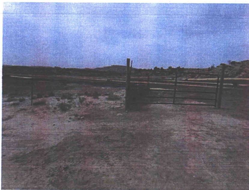
Photo 11 Three Strand Barbed Wire Fence and Site Gate
