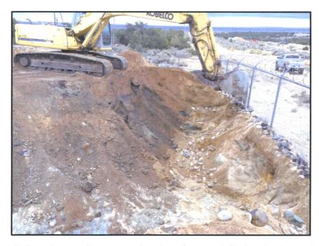
Figure 2. Excavation extending to west and southwest for removal of hydrocarbon impacted soils.
