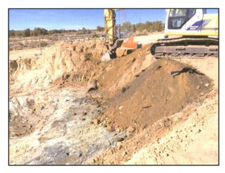
Figure 8. Excavation activities along the northern portion of the release location.
