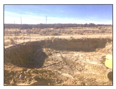
Figure 5. Southern extents of the excavation. Depth at sandstone ranged from 4-8 feet in the southern portion of the excavation.
