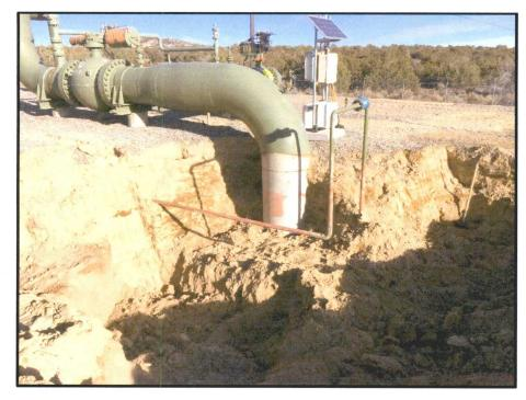
Figure 4. Continued excavation at the 2" header drip line and 30" suction line.
