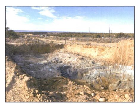
Figure 10. View to southwest of the final excavation. Size of excavation was approximately 72 feet by 37 feet, and ranged from 4 - 15 feet depth.
