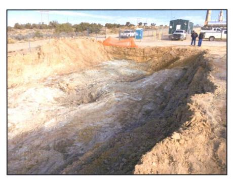
Figure 9. Northern extents of the excavation. Depth at sandstone ranged from 6-15 feet in the northern sections of the excavation.
