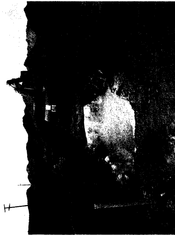
Trackhoe mixing contamination with Elke Solidification Product.
