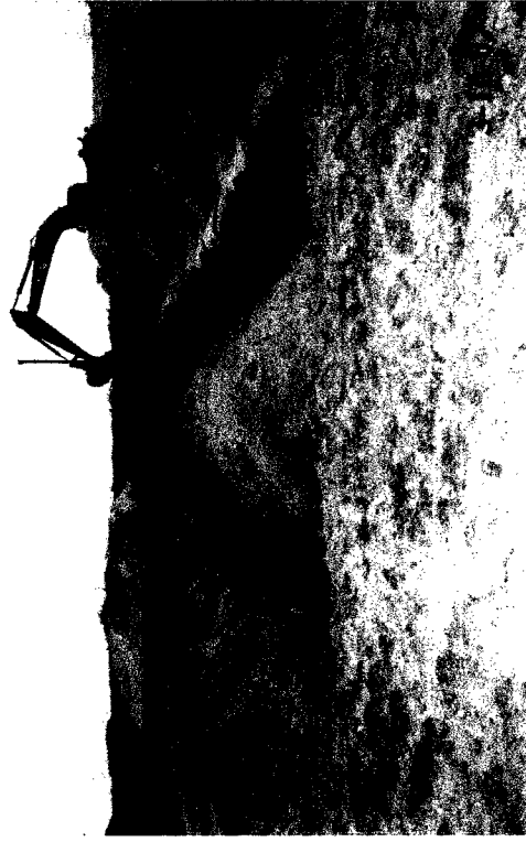
Placing solidified mud in burial pit.
