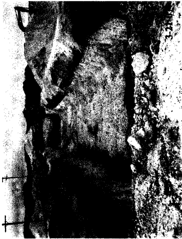
Excavation of second burial pit before liner.
