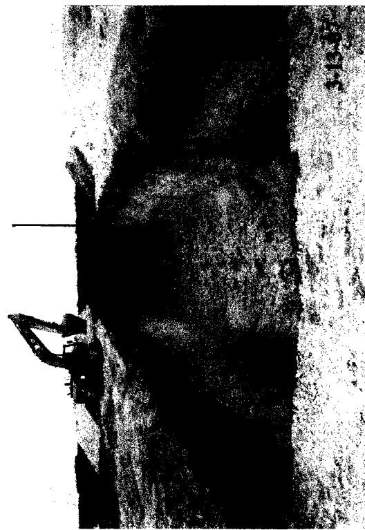
Excavation of burial pit before liner.
